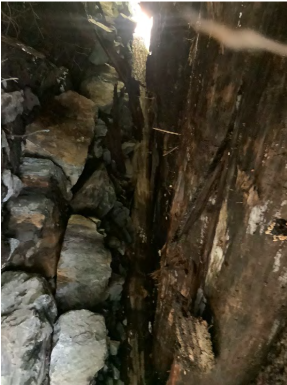
Left Bank Abutment when facing downstream
